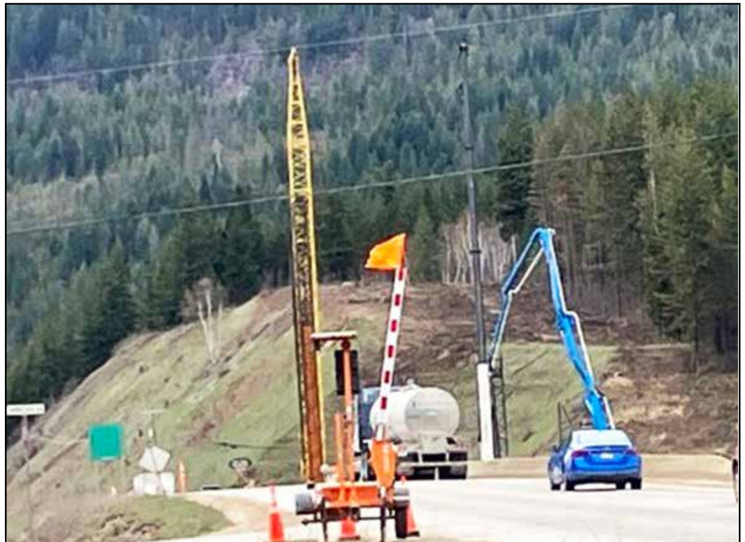
> Pile driving has begun on the new highway bridge in Tappen
