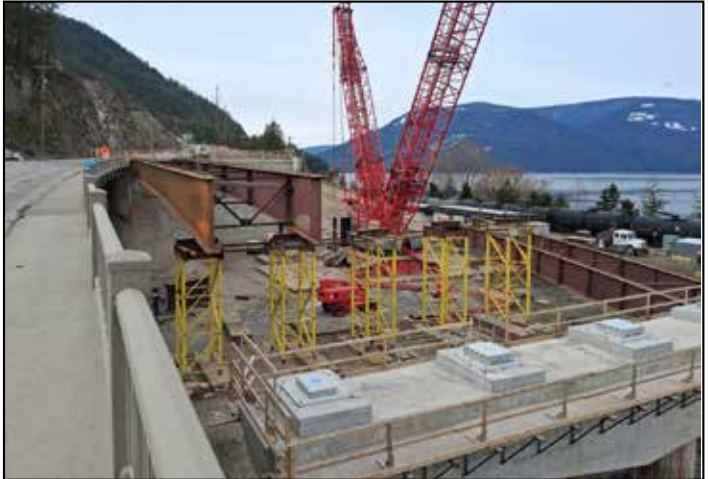
> Bruhn Bridge construction reached another milestone with the start of girder installations. Residents are advised they will hear a lot of clanking and grinding over the next three months.
